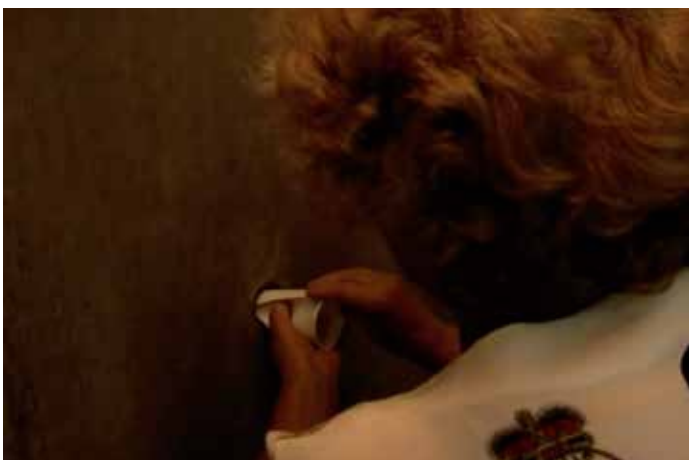
A leak is being tended to by inserting a cut plastic cup that better directs the flow of the water towards the bucket below, to not damage the wall.
