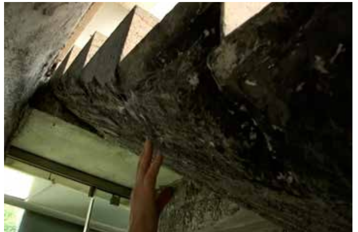
Explaining how the leaking and degradation of the iron and concrete are due to a section of the roof designed to be open.
