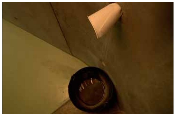
A leak is being tended to by inserting a cut plastic cup that better directs the flow of the water towards the bucket below, to not damage the wall.
