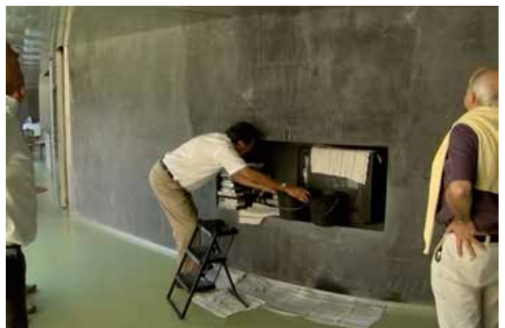
Rain water leaks tended to by collecting the water with buckets and towels.
